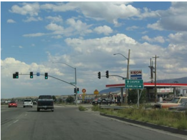
Figure 2. Intersection in Mills that was recently completed.
